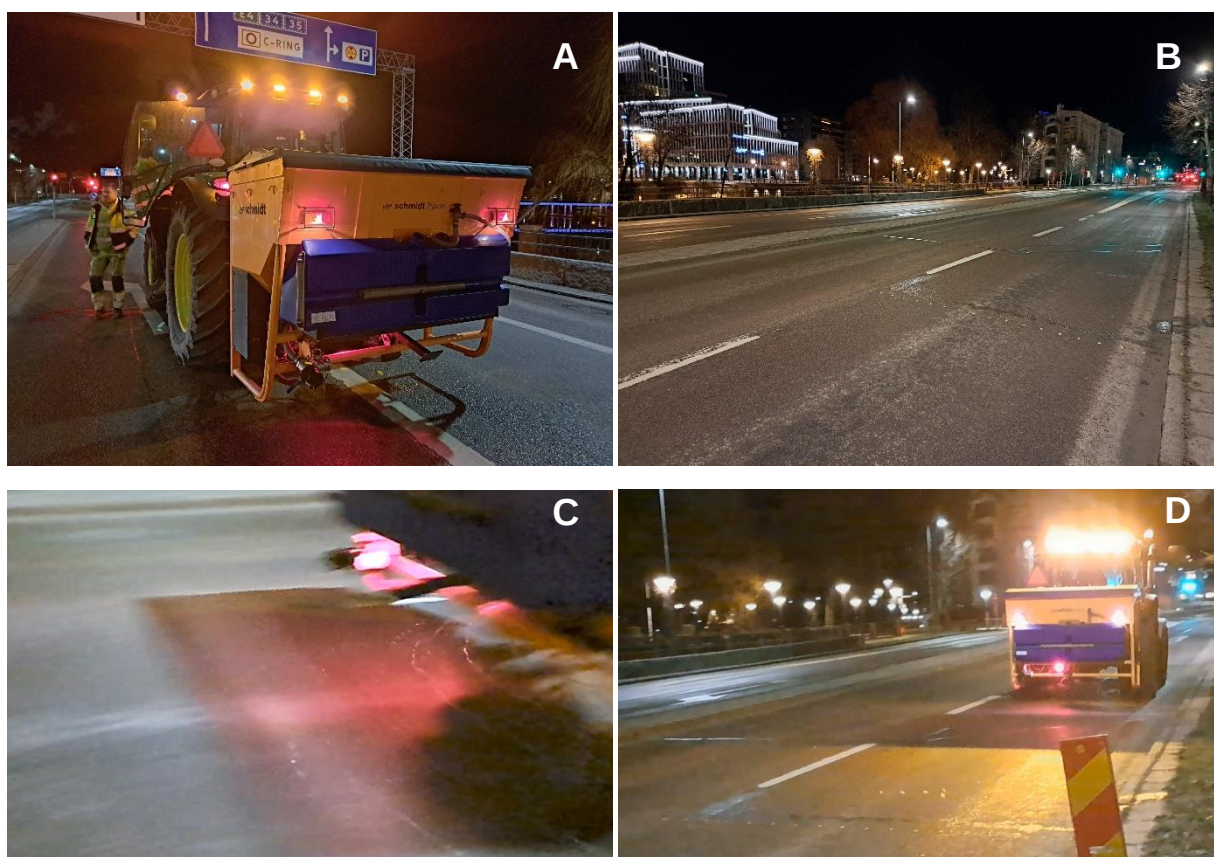
Figure 63. Application of CMA using a tractor with a tank and spinner disc (A). Resulting CMA deposition pattern (B). The spinner spreading CMA at the sampling site (C) and the tractor while applying CMA (D). Photos: Mats Gustafsson and Göran Blomqvist, VTI.
